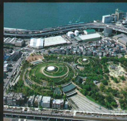
Osaka Municipal Central Gymnasium
